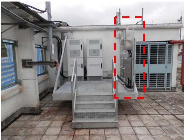
(b) BD confirmed that if split-type A/C condensers could be shared with the supporting structure for a radio base station if they solely served the radio base station.
